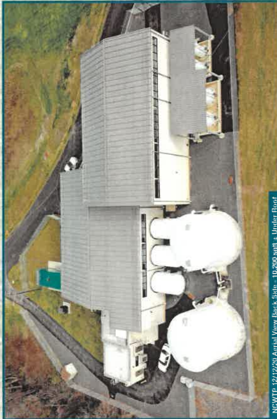
Radium Removal (4) Tanks
